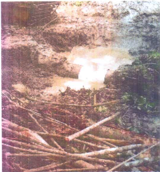
SPILL POINT AFTER REPAIR: fig3
