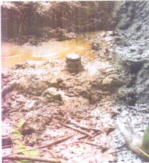
SPILL POINT AFTER EXCAVATION: fig1
